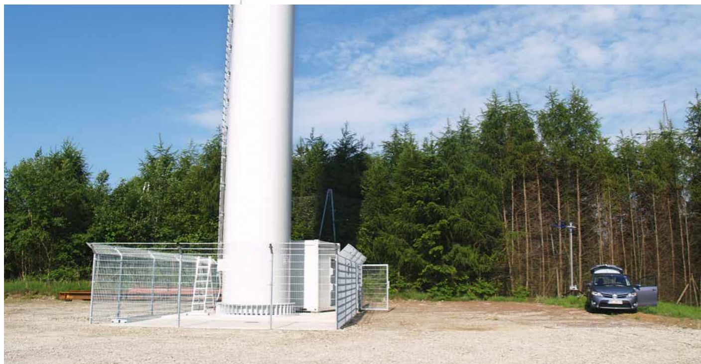
Test arrangement „radio interference strength measurement“
