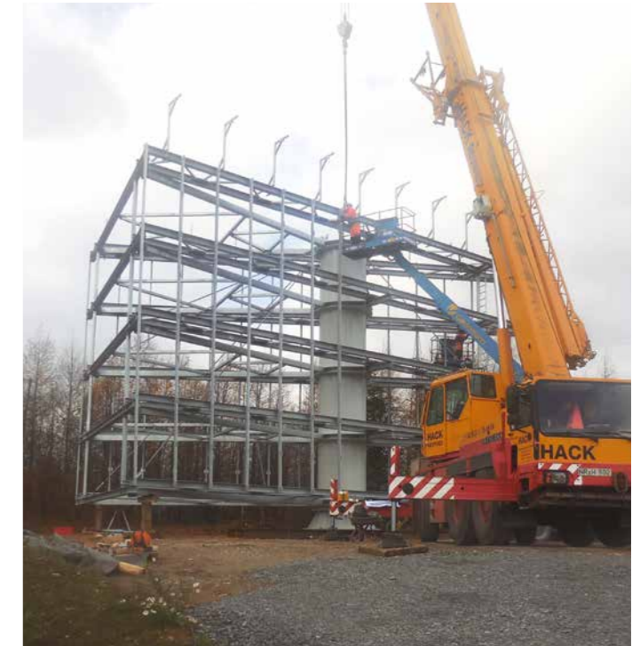
30 t steel work
